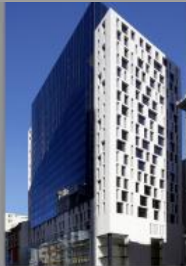
77 King Street Office Tower, Sydney
