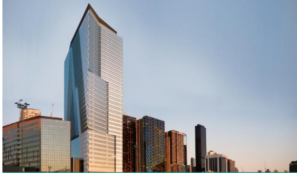
Topped out 311 Spencer Street in Melbourne
